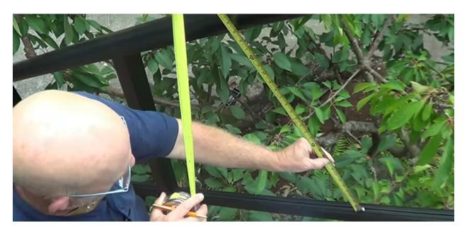
**Step 18** - To obtain the right offset dimension, place your square parallel with the bottom rail and up against the right post. Measure from the face of the right post to the edge of your square to obtain the right offset dimension, and record your measurement under RO.
