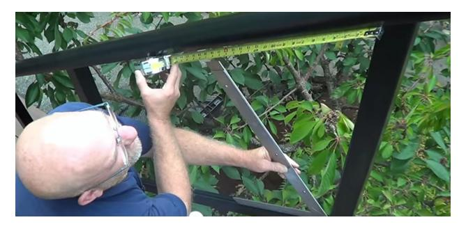
**Step 19** - The same process is used to obtain the left offset measurement, except the square is placed parallel with the top rail. Record your measurement under LO.
