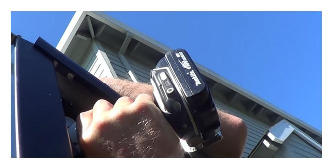
**Step 8** - Install the end plates with the stainless steel sheet metal screws.
