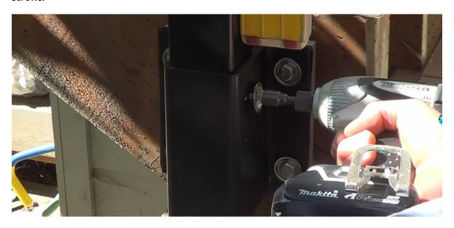
**Step 4** - Install the top rail brackets on the top and bottom posts.
