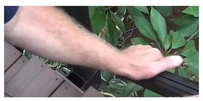
**Step 16** - Start measuring the glass by measuring the horizontal distance from post to post, just under the top rail. Record that measurement at B, then deduct three inches to arrive at the net glass width.
