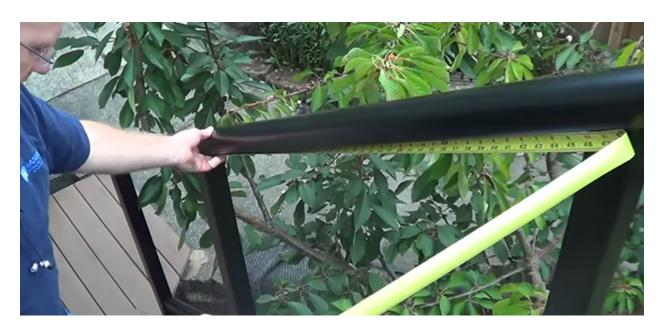
**Step 17** - Then take a perpendicular measurement on the height and put it on the H measurement. Add 3/4" to the height measurement to arrive at the net height.
