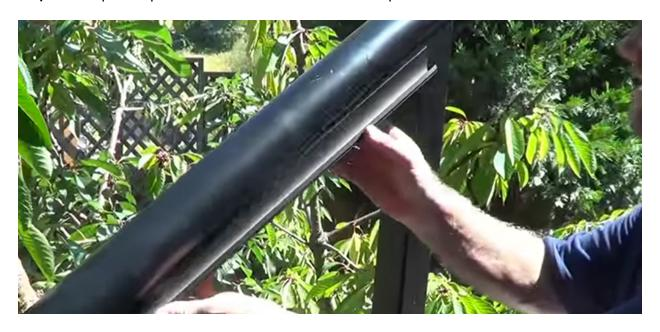
**Step 14** - Snap the bottom rail over the top of the connecting blocks.
