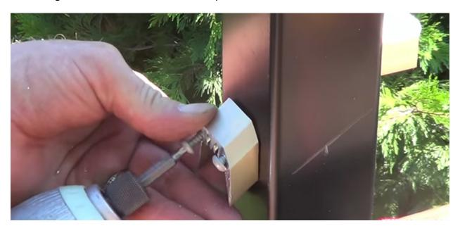
**Step 11** - Using a string line, measure the intermediate posts and mount the railing connecting blocks.
