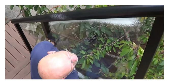
**Hint** - Use a little glass cleaner to lubricate the glass to aid in the installation.
