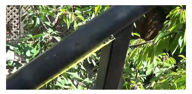
**Step 13** - Snap the top rail infill into the underside of the top rail
